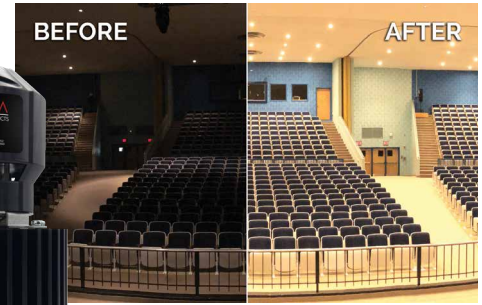
Fairfax High School, Fairfax, Virginia 105 RETRO 500s at 3000K Installed by Artistic Concepts Group
